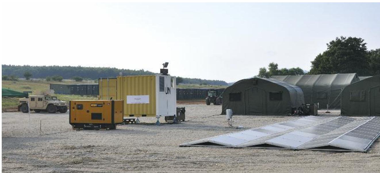
ESTechnologies Smart Energy plant during CL15
